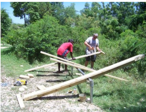
Play ground repairs
