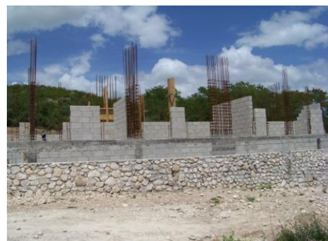
West side of the building looking east
