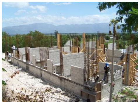
Back of the health center looking northwest
