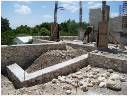
Front of the building handicap accessible ramp under construction
